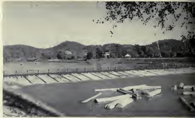
RICE RAFTS made of teakwood float right over the spillway of the diversion dam on the Me Ping River in northern Siam. This is part of the Me Fact project, 16 years old, serving about 40,000 acres, and providing much of Siam's most important crop—rice, plus many other substantial benefits.
